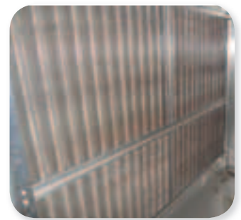
details of the droplet separator
