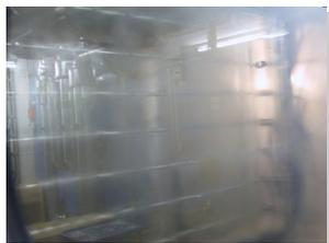
The sprayed water is supplied by a reverse osmosis treatment system so that the maintenance of the humidifier is strongly reduced. The humiFog pumping station is equipped with a Variable Frequency Driver and a multi stage atomising technology obtaining a wide modulation range: the BMS can require humiFog any flow rate in the range 47 to 246 kg/h. In this way, humiFog will spray exactly and only the quantity of water the BMS is requiring.
